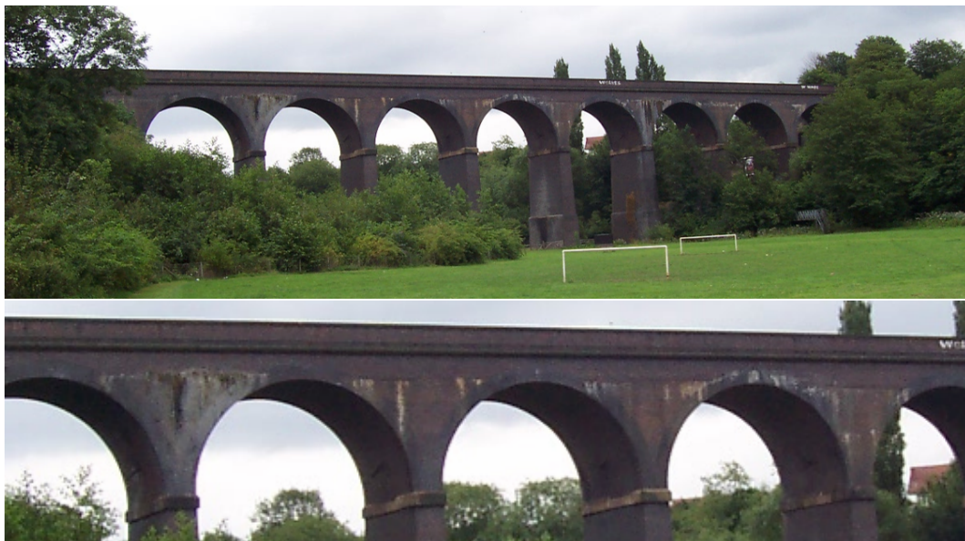
Figure E.3: Photographs of Example 2 bridge
