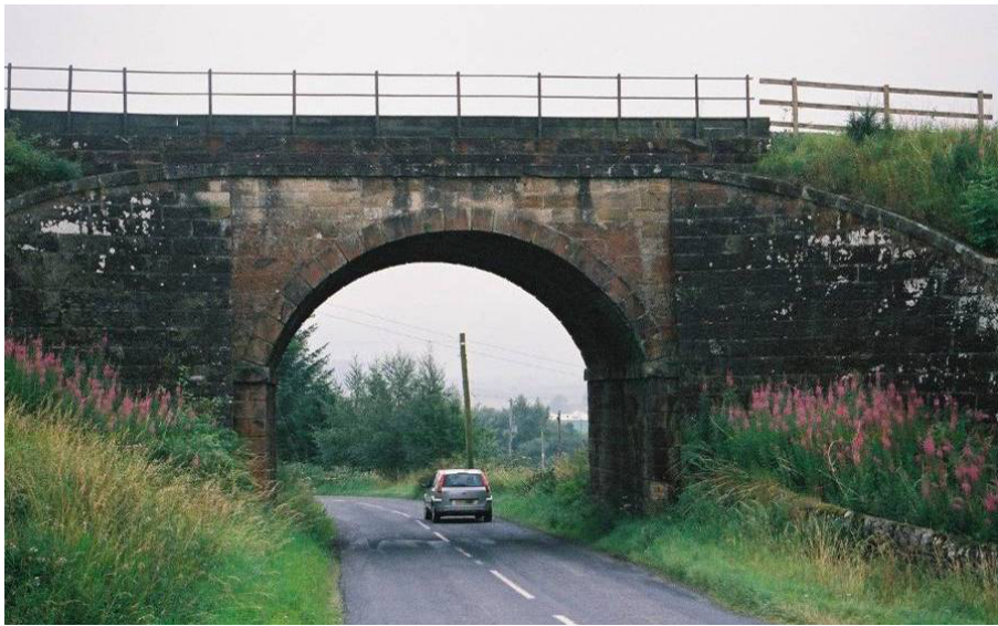
Figure E.1: Photograph of Example 1 bridge
