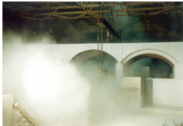
Figure G.4: Bolton bridge Multi-2 immediately following collapse (note that the right span has remained fully intact)
