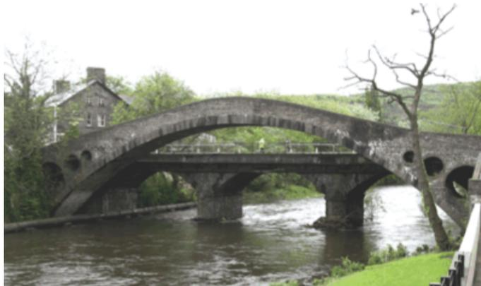
Figure 2: Williams' bridge at Pontypridd, showing spandrel voids
